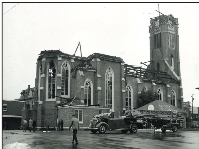
Exterior of the fire damage to the old Saint Boniface Church in Williamsport, after flames swept through the 97-year-old structure on Dec. 5, 1972. (Photo/The Catholic Light archives)
