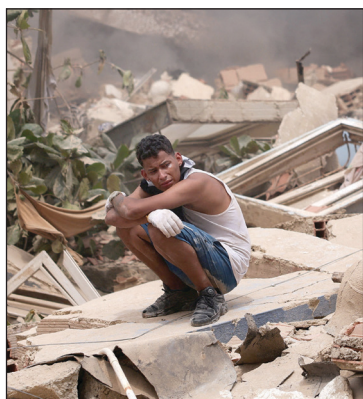
A young man reacts amid the rubble of a destroyed building in La Guaira, Venezuela, June 25, 2026, following 7.2 and 7.5 magnitude earthquakes that rocked the country June 24. (OSV News photo/Gaby Oraa, Reuters)
